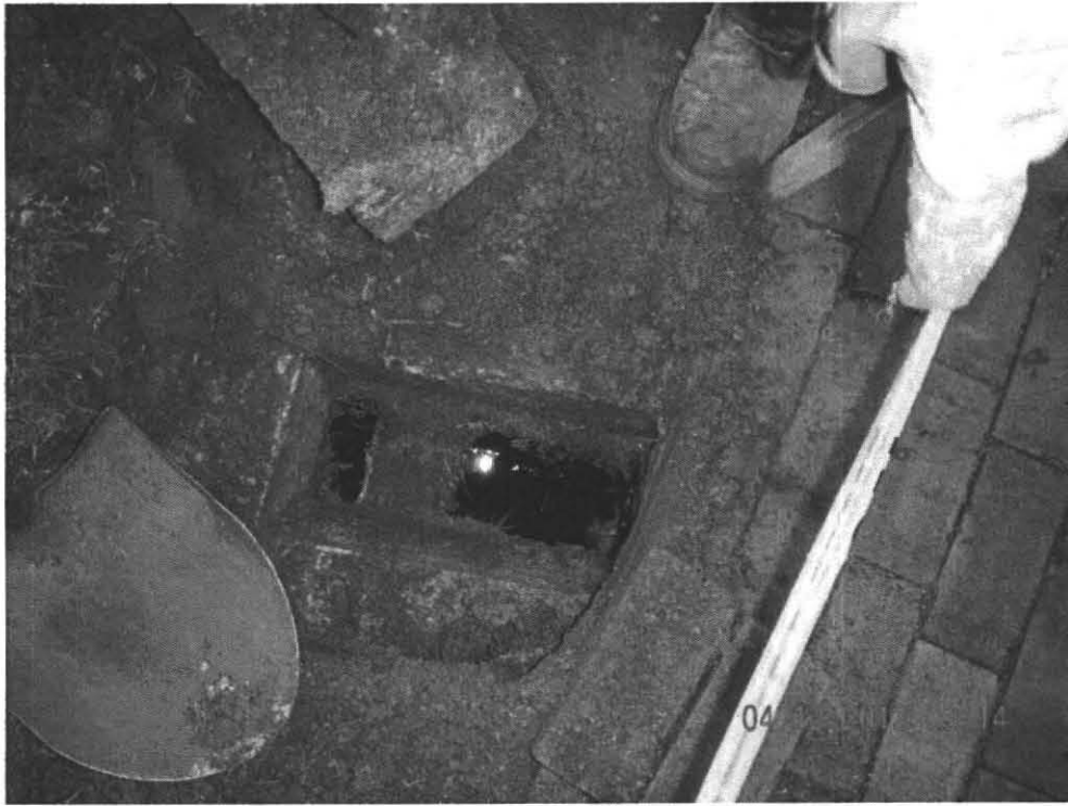
S. Tank Inlet Baffle pipe 35 Trillium Way Amherst, MA 04.12.2013
