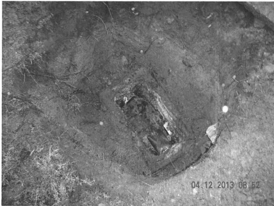
D. Box (heavy biosolids, half in pipe) 35 Trillium Way Amherst, MA 04.12.2013
