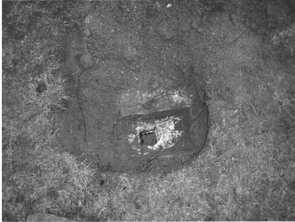
S. Tank Outlet Baffle pipe 35 Trillium Way Amherst, MA 04.12.2013
