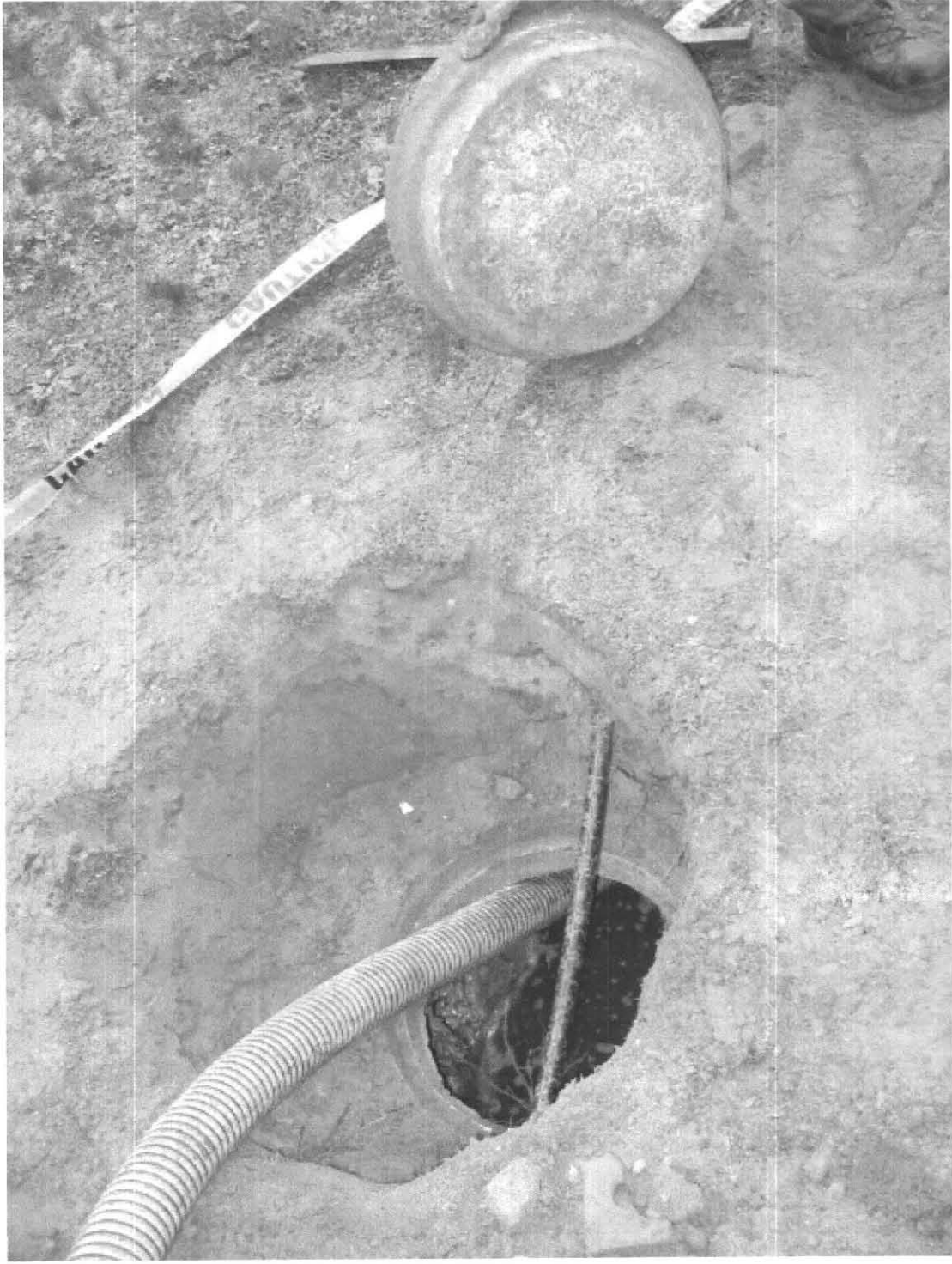
Septic Tank 18 Trillium Way , Amherst, MA 06.04.2008
