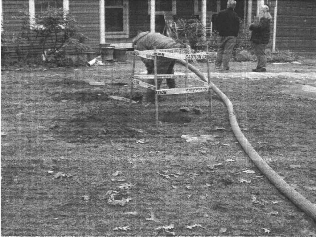
Septic Tank Area 7 Trillium Way Amherst, MA 02.02.2012
