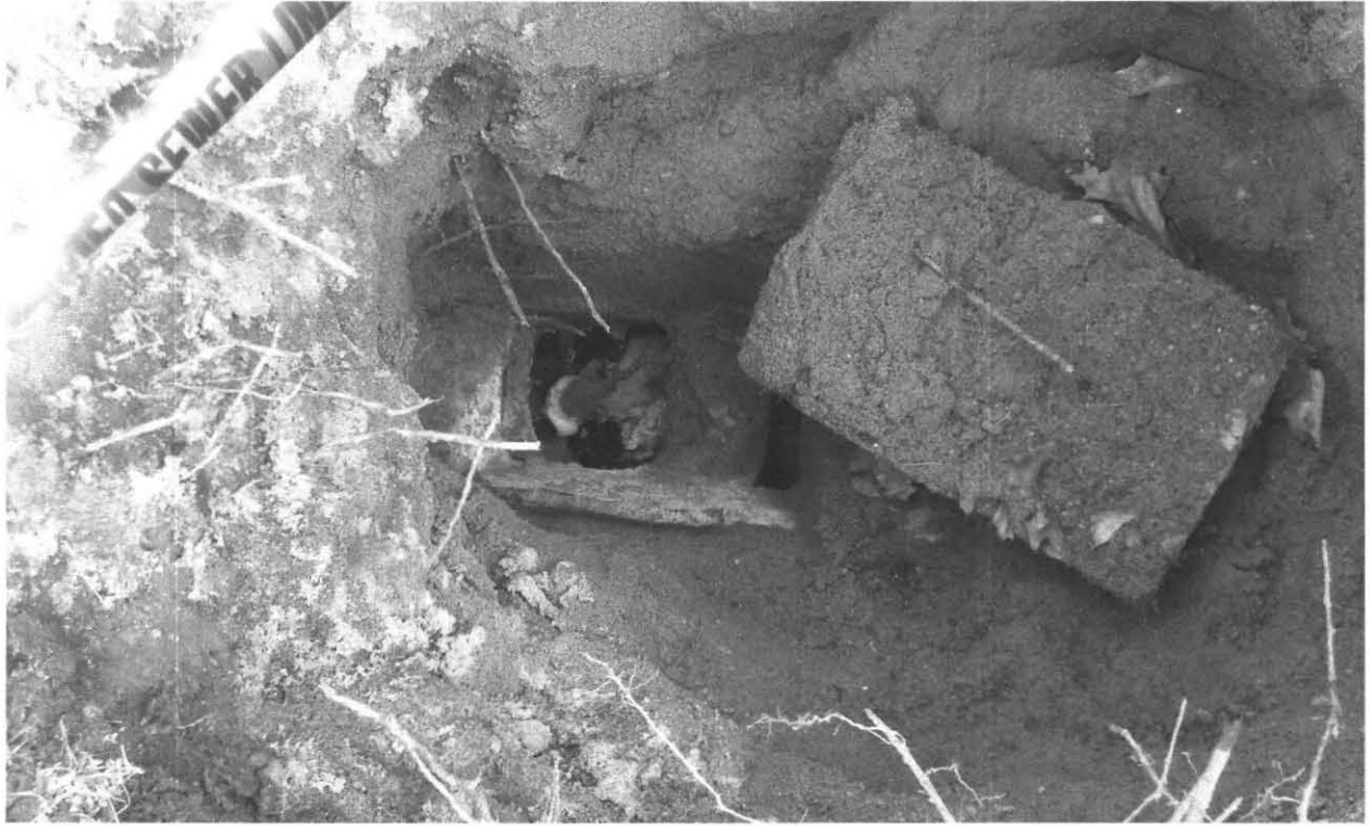
S. tank Inlet Baffle. 23 Teaberry Lane Amherst, MA 03.25.2010
