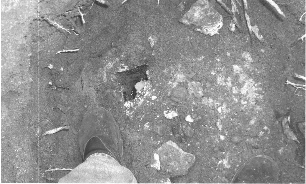
Old Dist. Box (Replaced) 23 Teaberry Lane Amherst, MA 03.25.2010
