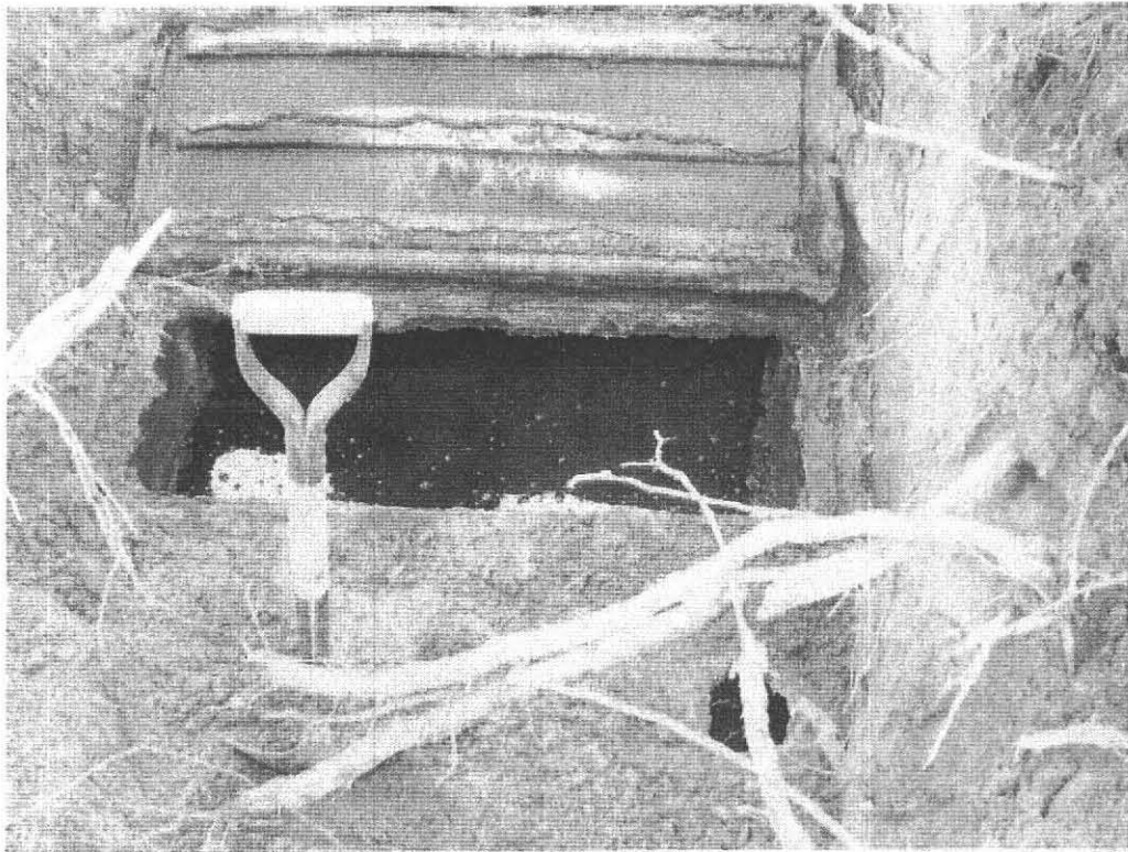
Arc Type Septic Tank 456 Sunderland Road Amherst, MA 12.22.2011
