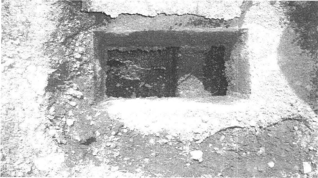
Inlet Baffle 677 Station Road Amherst, MA 06.08.2010
