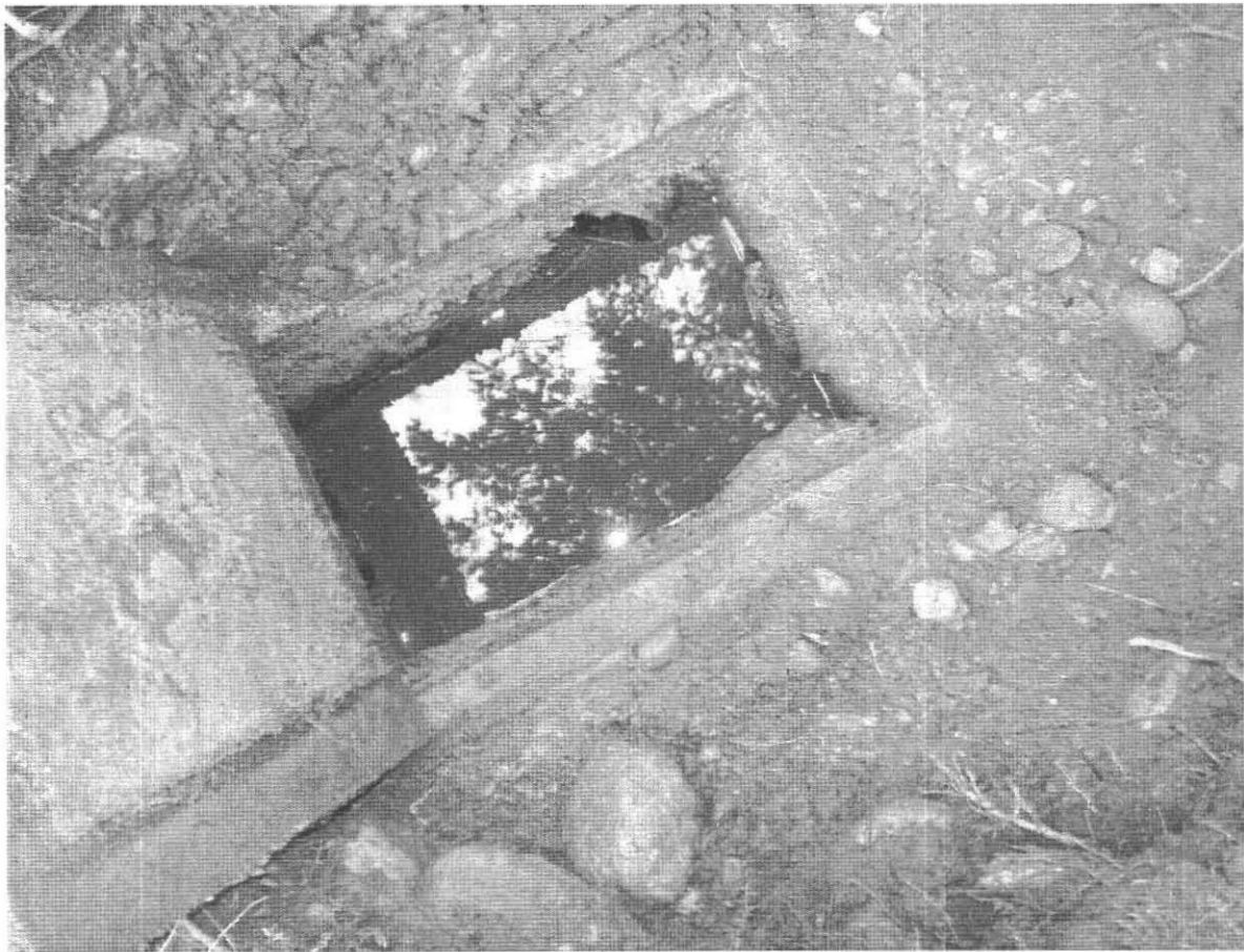
D. box (old) cracked 418 State Street Amherst, MA 05.16.2012
