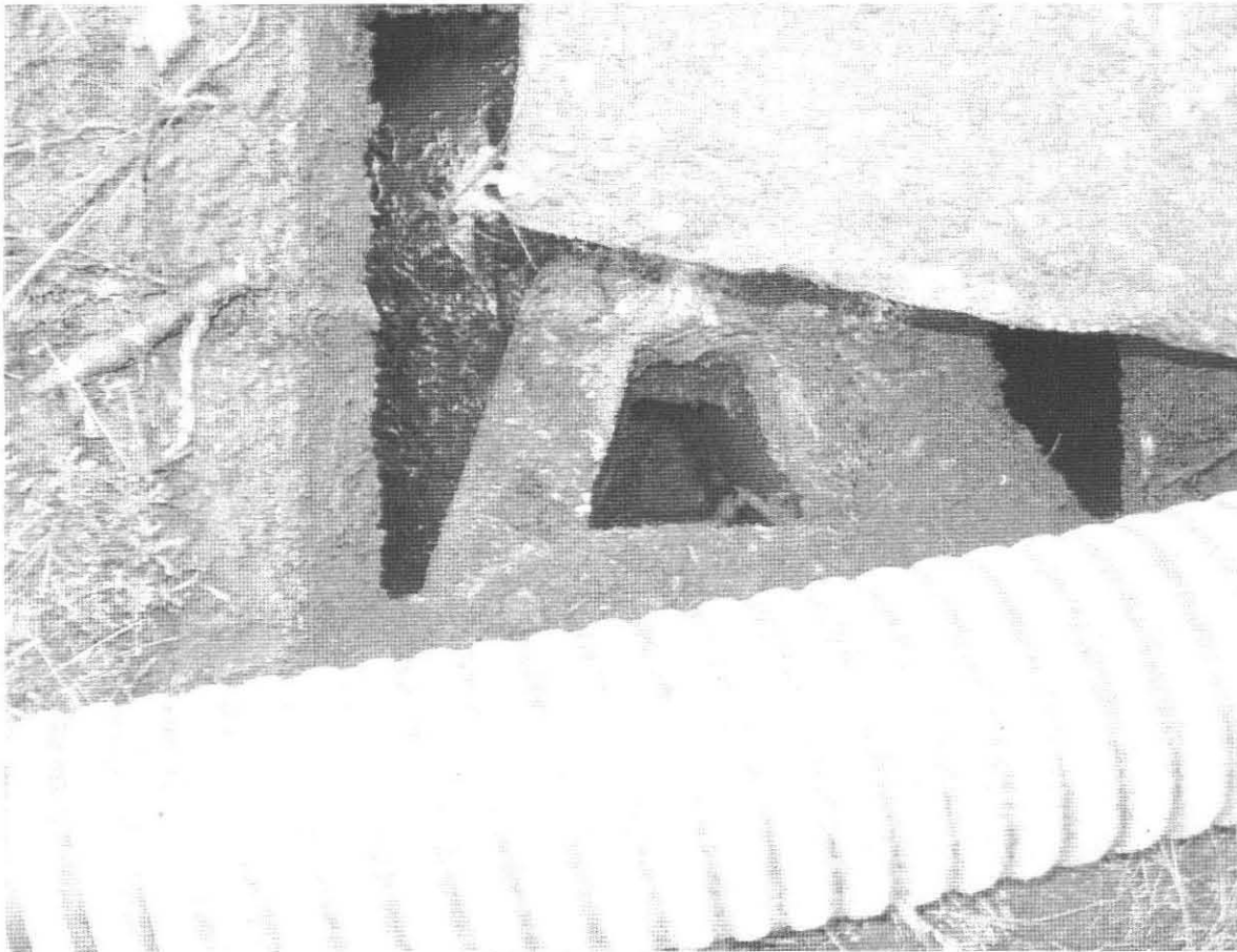
S Tank Outlet Baffle 418 State Street Amherst, MA 05.16.2012
