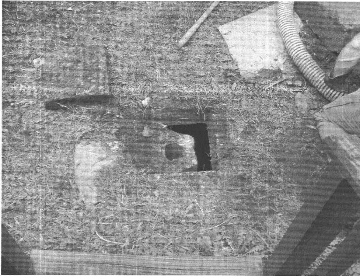
S Tank Inlet Baffle 418 State Street Amherst, MA 05.16.2012
