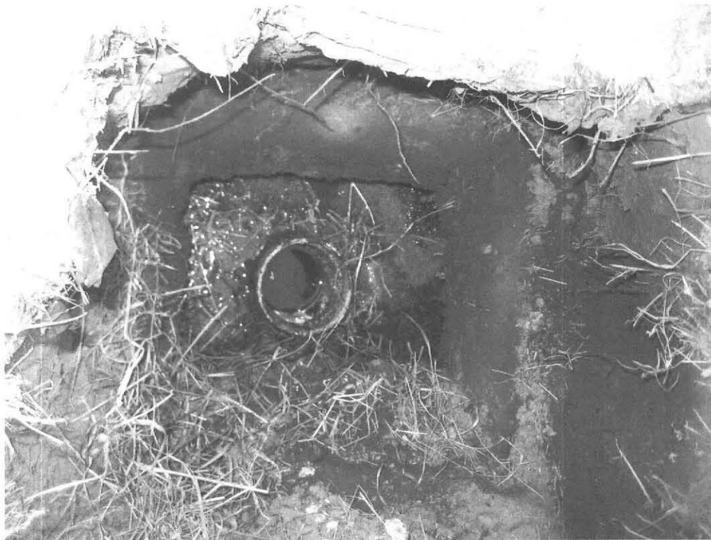
S. tank Outlet tee 76 stagecoach Road Amherst, MA 12.23.2009
