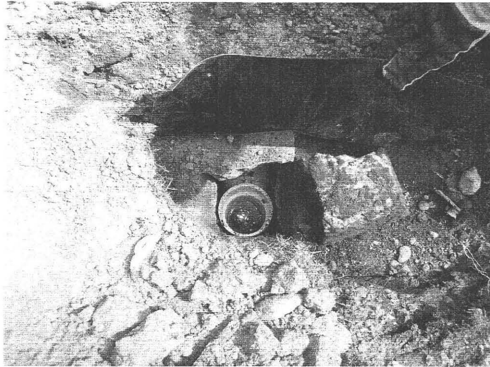
New Outlet tee from S. Tank 307 Shutesbury Road Amherst, MA 04.11.2011
