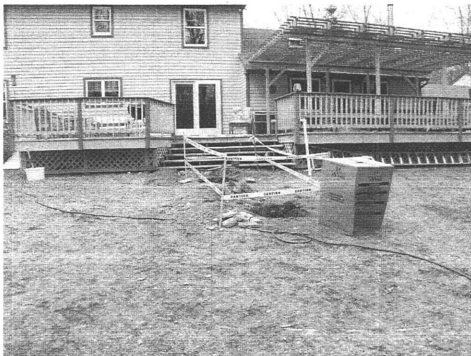
Septic Location 307 Shutesbury Road Amherst, MA 04.08.2011
