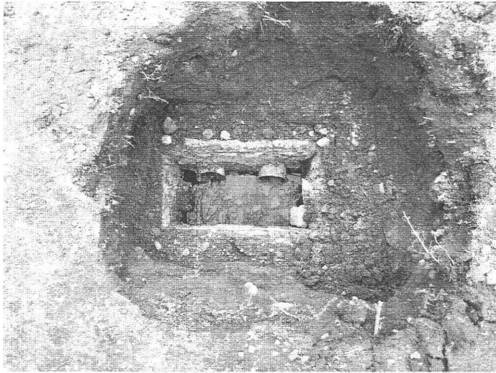
Old Replaced Corroded Dist. Box 307 Shutesbury Road Amherst, MA 04.08.2011
