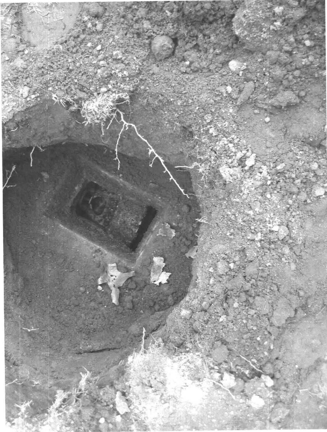
Tank Outlet baffle 297 Shutesbury Road Amherst, MA 04.01.2009
