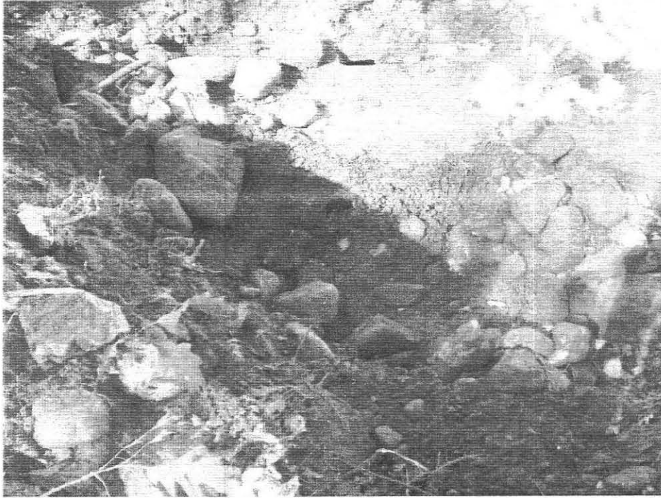
Dry well 330 Pelham Road Pelham, MA 11.01.2011
