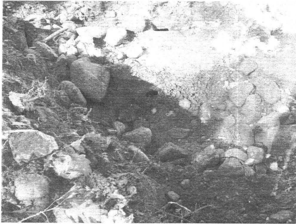
Dry well 330 Pelham Road Pelham, MA 11.01.2011
