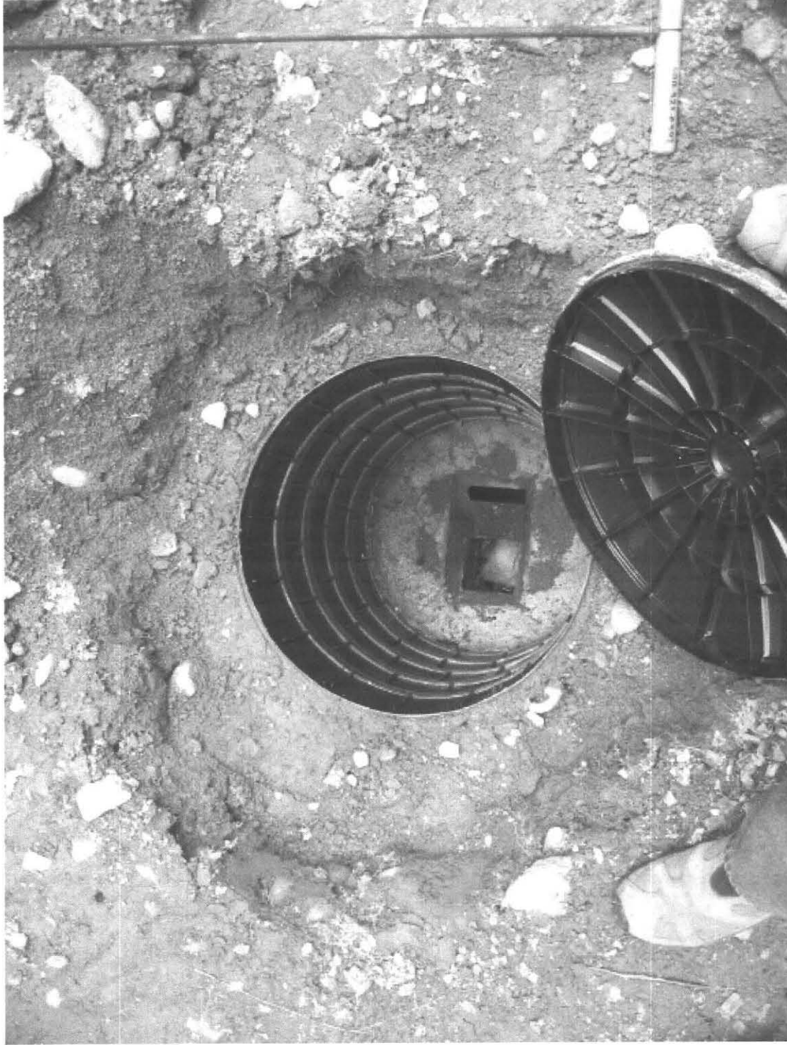
Septic Tank Baffle 66 Overlook Drive Amherst, MA 07.31.2008
