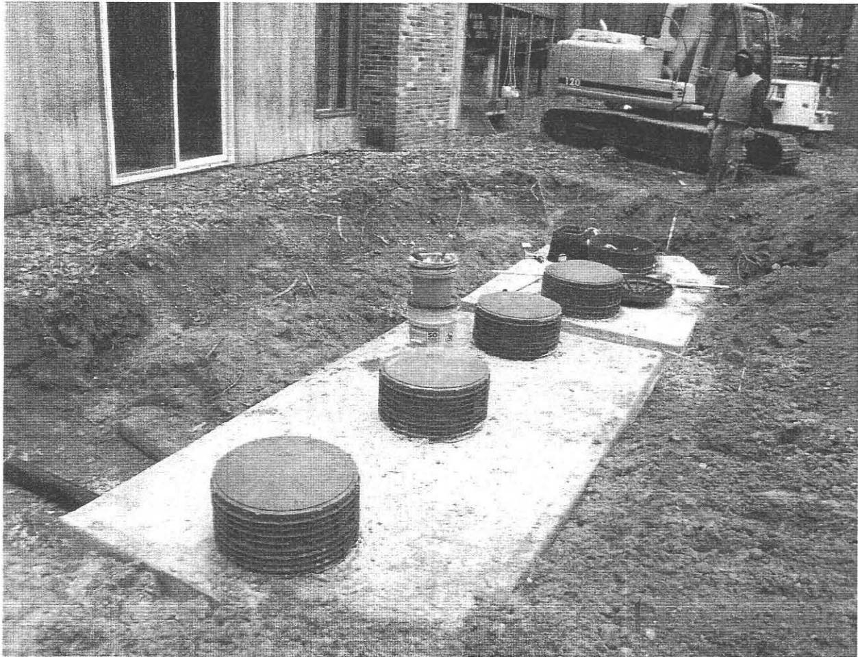
New S. tank and P. Chamber 11 Overlook Drive Amherst, MA 11.02.2010
