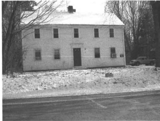
Deep holes and perc test for 273 Montague Road 12/5/07
