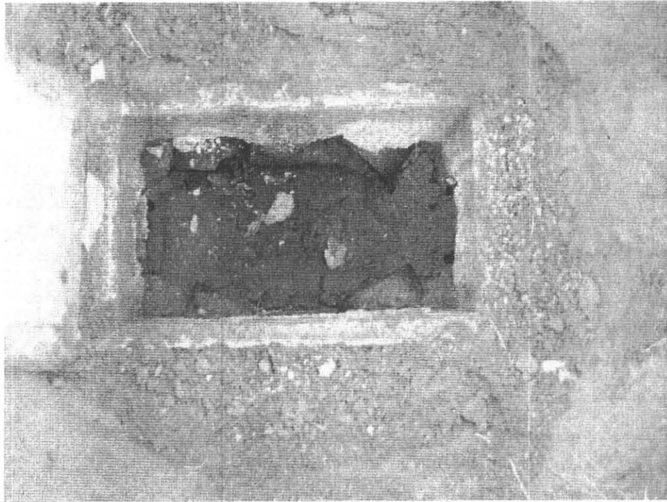
Sludge in Dist. Box 237 Meadow Street Amherst, MA 12.22.2011
