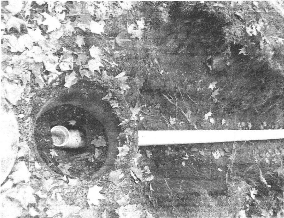
Repaired line to (inlet tee) at S. tank at Whirlwind Kennels 435 Market Hill Road Amherst, MA 10.19.2010
