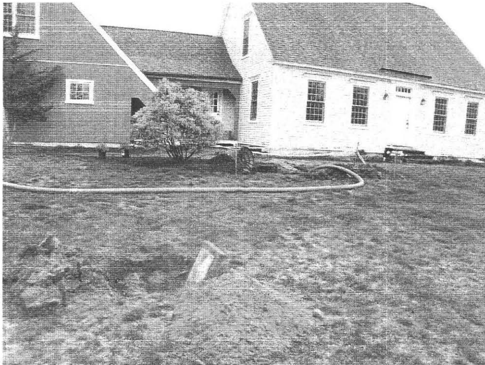
Septic System Area 305 Leverett Road Amherst, MA 04.19.2011
