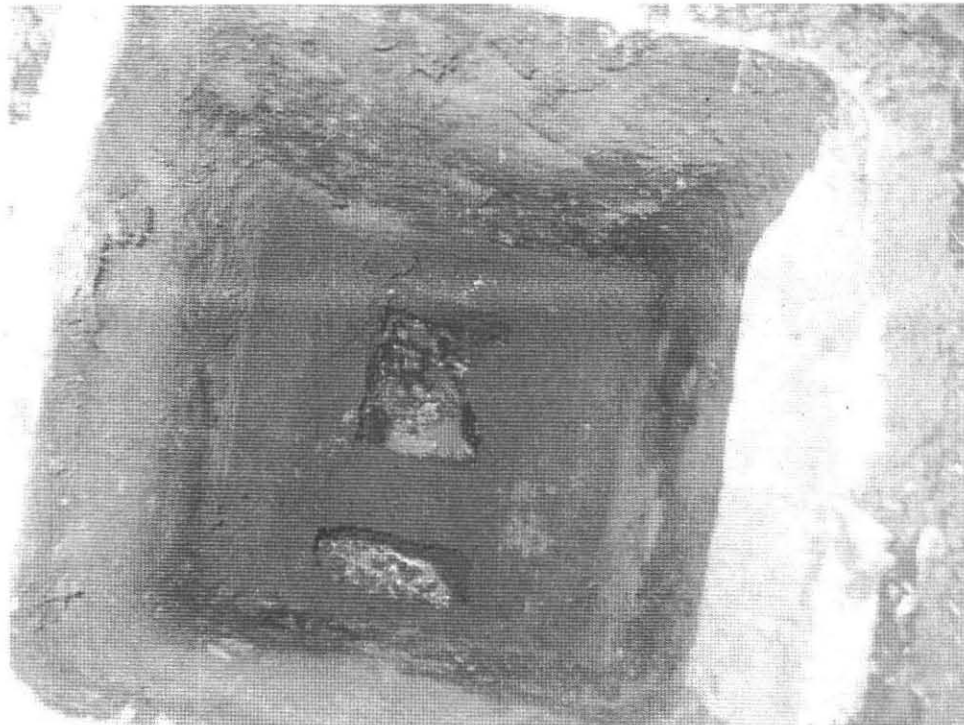
S. Tank Inlet Baffle 115 Levertt Road Amherst, MA 06.01.2012
