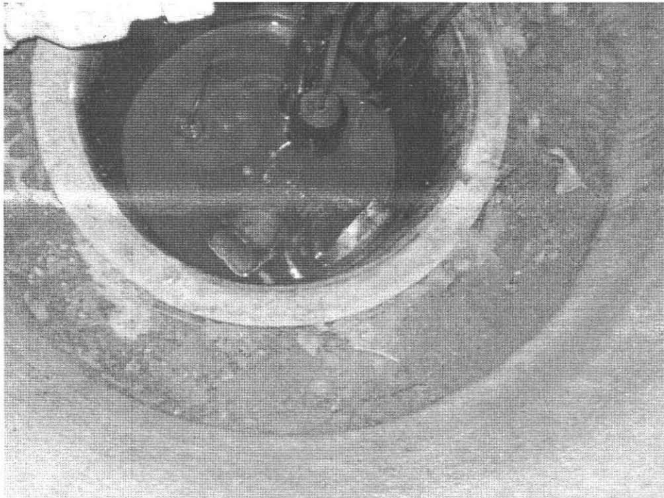
Pump & Chamber 115 Levertt Road Amherst, MA 06.01.2012
