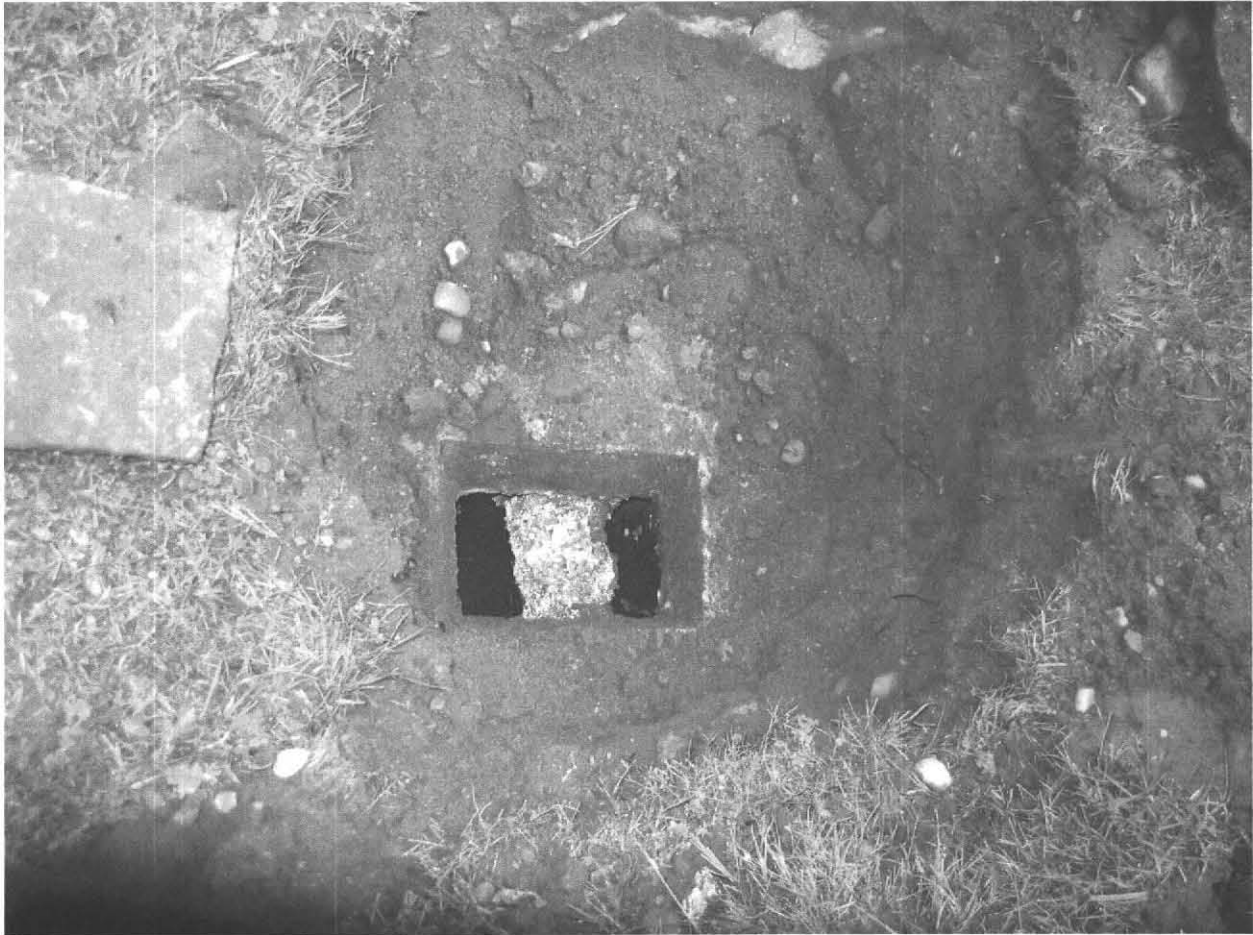
Septic Tank Outlet 7 Ladyslipper Lane Amherst, MA 05.27.2009
