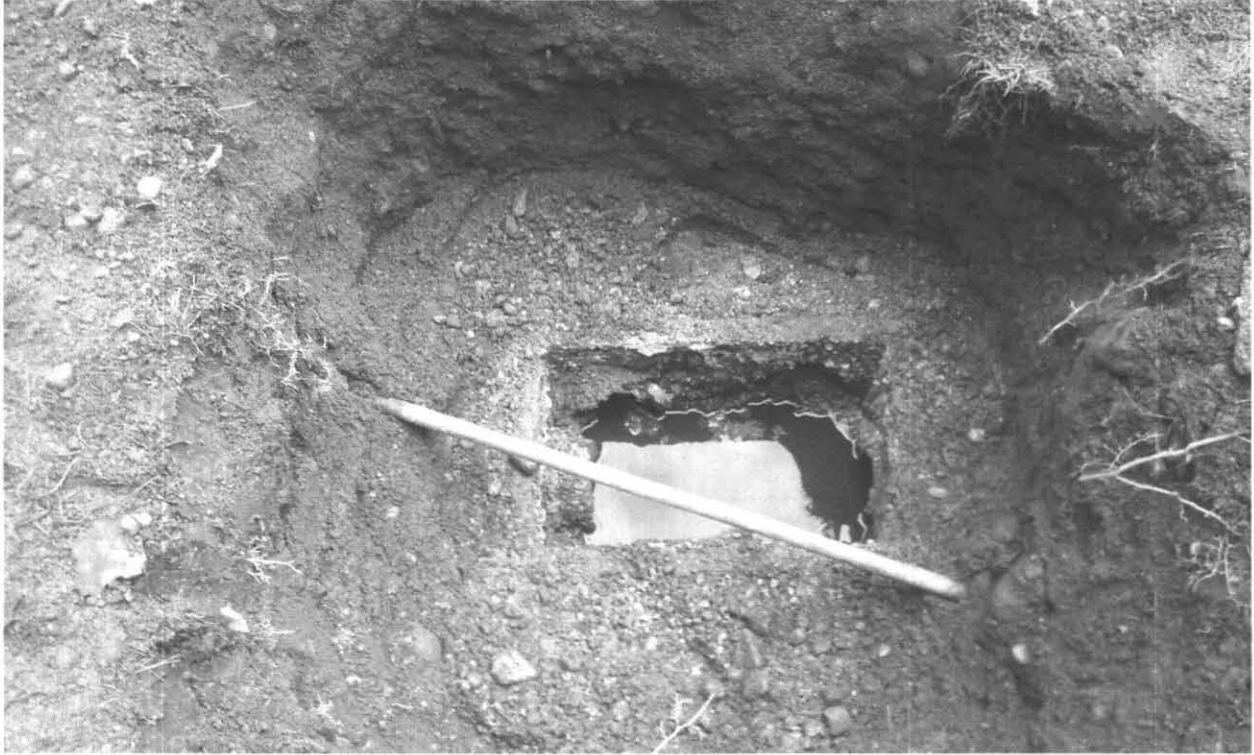
Dist Box Corroded, (saturation over inverts) 21 Highpoint Drive Amherst, MA 03.24.2010
