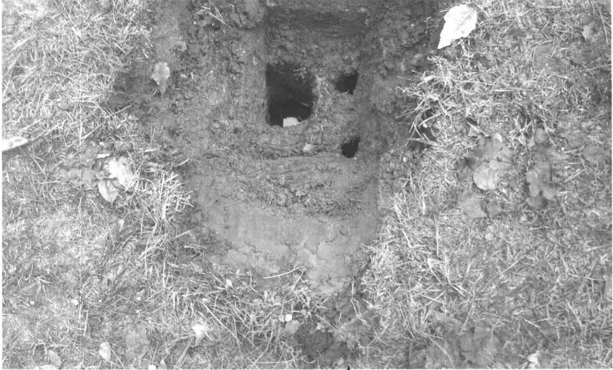
S. Tank outlet Baffle Cover, 21 Highpoint Drive Amherst, MA 03.24.2010
