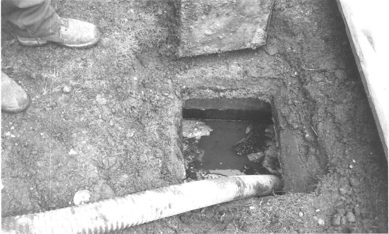
S. Tank Cover, (Inside staining, past) 21 Highpoint Drive Amherst, MA 03.24.2010
