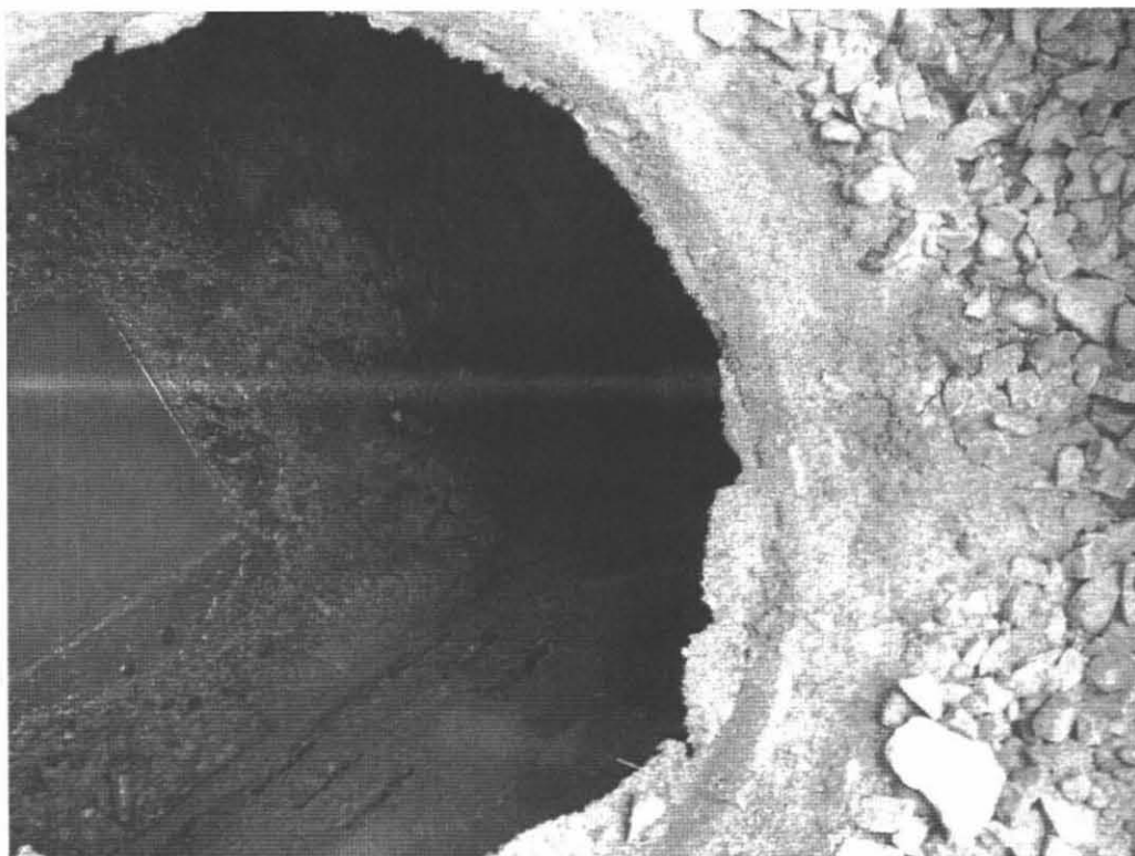
Leaching Tank 16 Foxglove Lane Amherst, MA 04.05.2012
