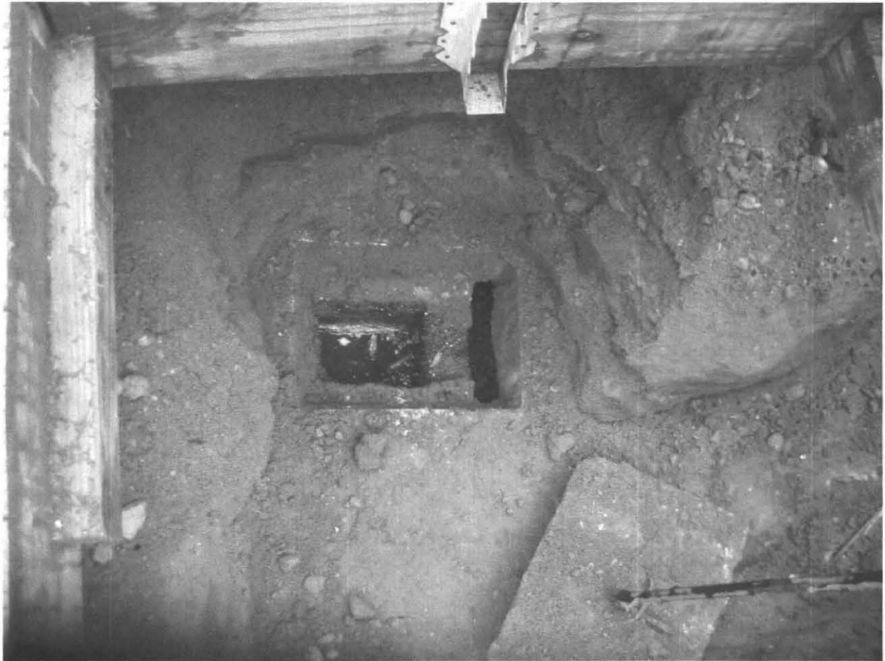
Septic Tank Inlet, under Deck 15 Foxglove Lane Amherst, MA 05.27.2009
