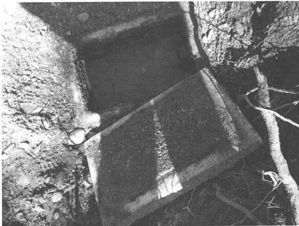
Failed Dist. Box 66 Flat Hills Road Amherst, MA 03.20.2012
