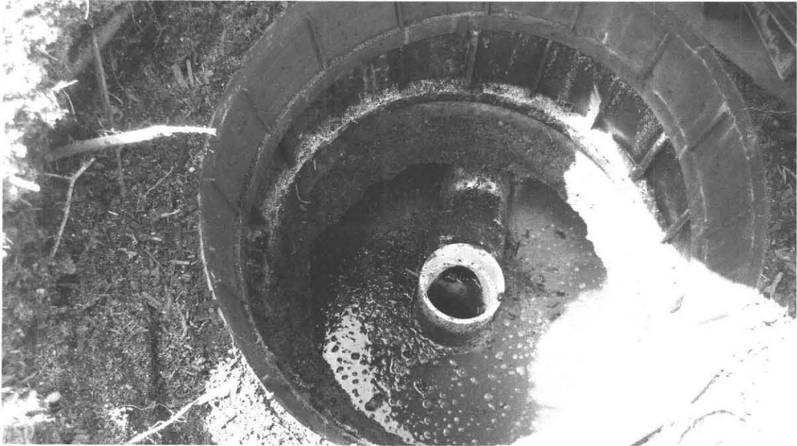
S. Tank Outlet 23 Dayton Lane Amherst, MA 04.20.2010
