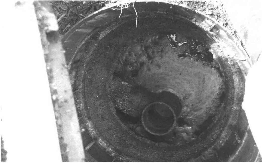
S. Tank Inlet 23 Dayton Lane Amherst, MA 04.20.2010
