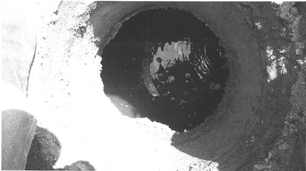
L. tank Prior to stone repair 20 Bridal Path Amherst, MA 04.20.2010
