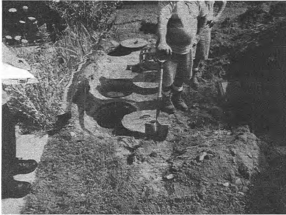
S. Tank and D. Box cover 670 Bay Road Amherst, MA 7.19.2011
