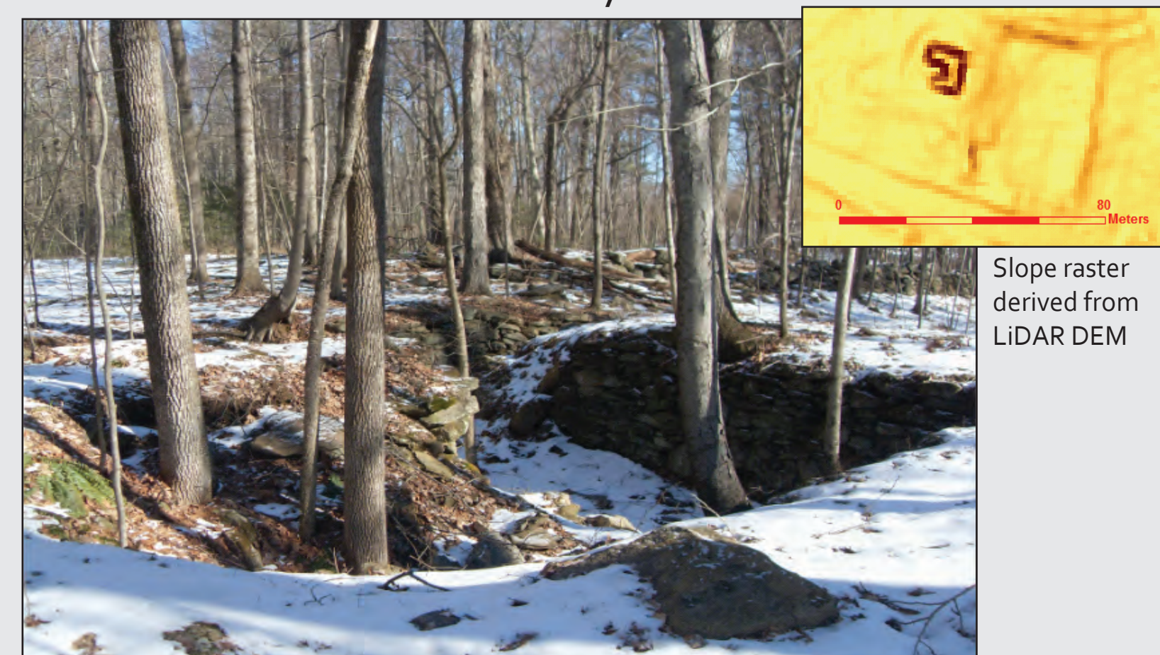
Photograph of foundation as seen in field
